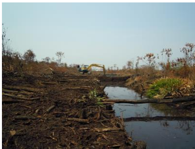
Check-dam/canal blocking constructed using heavy machinery to raise the water level at the pilot site
