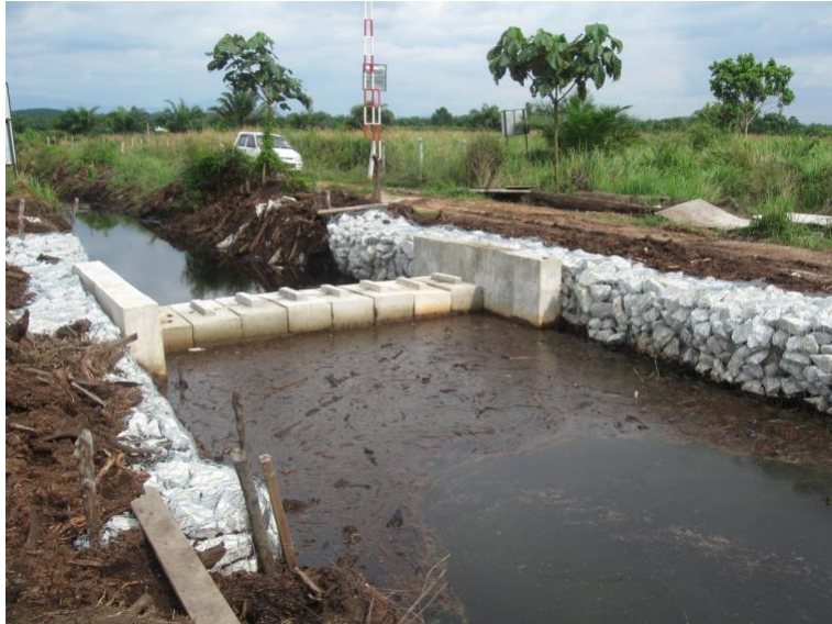
Concrete check-dam constructed under APFP
