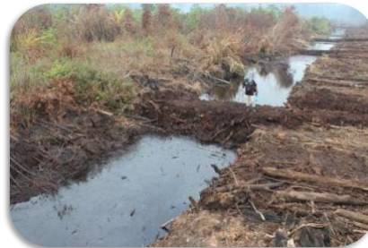
Check-dam/canal blocking constructed using heavy machinery to raise the water level at the pilot site
