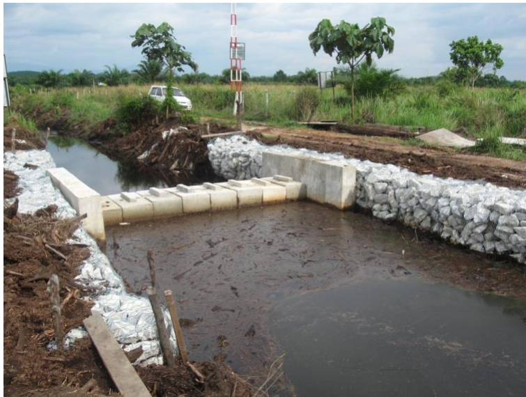
Concrete check-dam constructed under APFP
