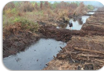
Check-dam/canal blocking constructed using heavy machinary to raise the water level at the pilot site
