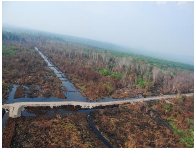
Clay bund constructed by PKPS to raise the water level at the fire prone area
