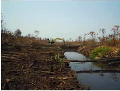
Check-dam/canal blocking constructed using heavy machinary to raise the water level at the pilot site
