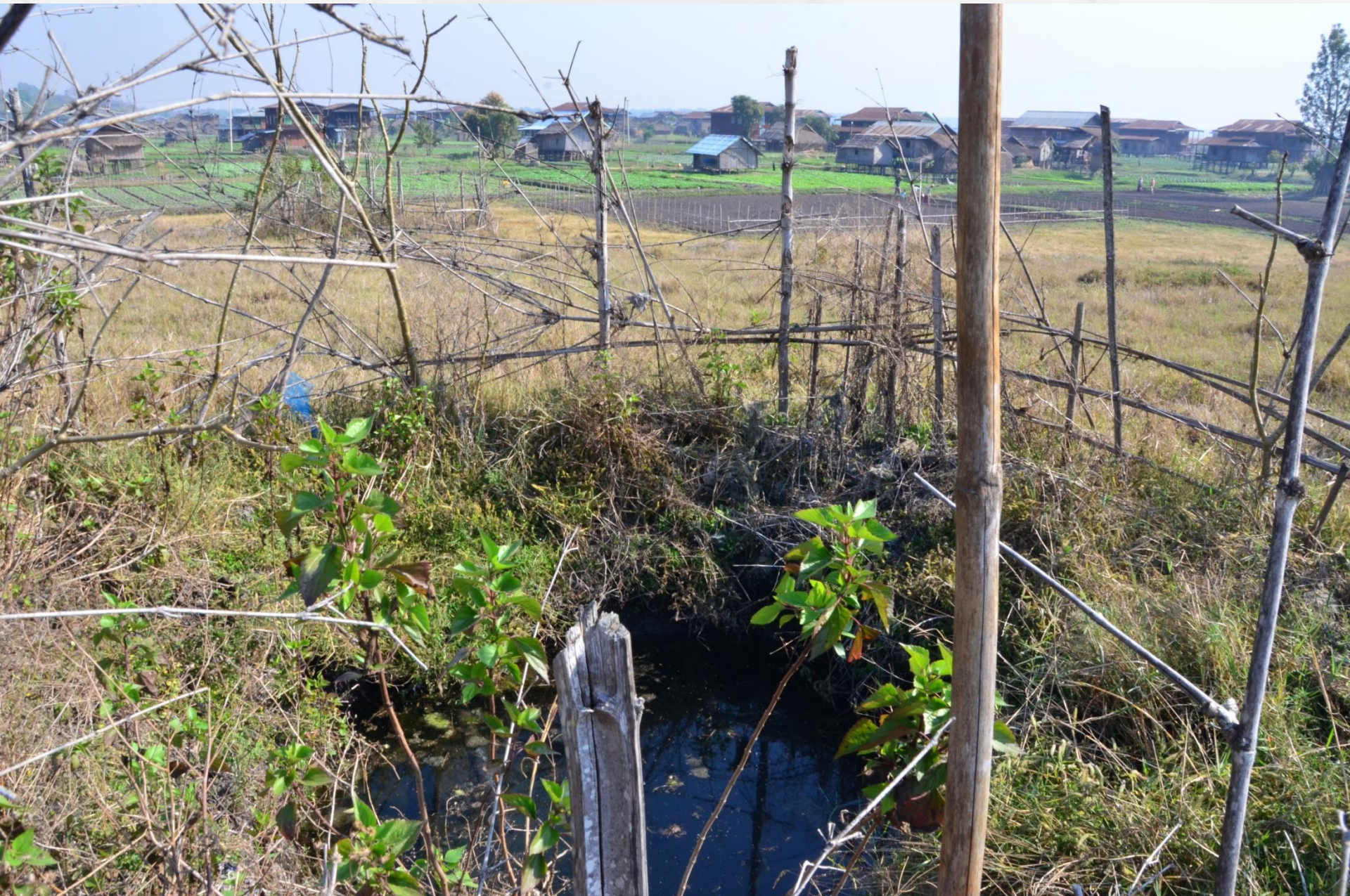
Open well cut by villagers connected by pipes to selected houses.
